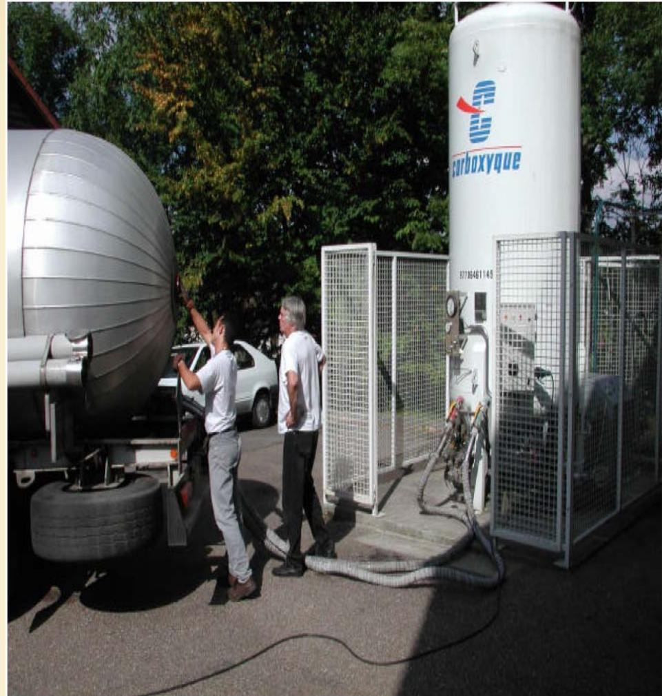
Carbon dioxide supply to SEPAREx tank (4 tonnes) from a cryogenic truck
